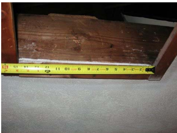
An example of an attic scuttle hole that requires evaporator disassembly.
