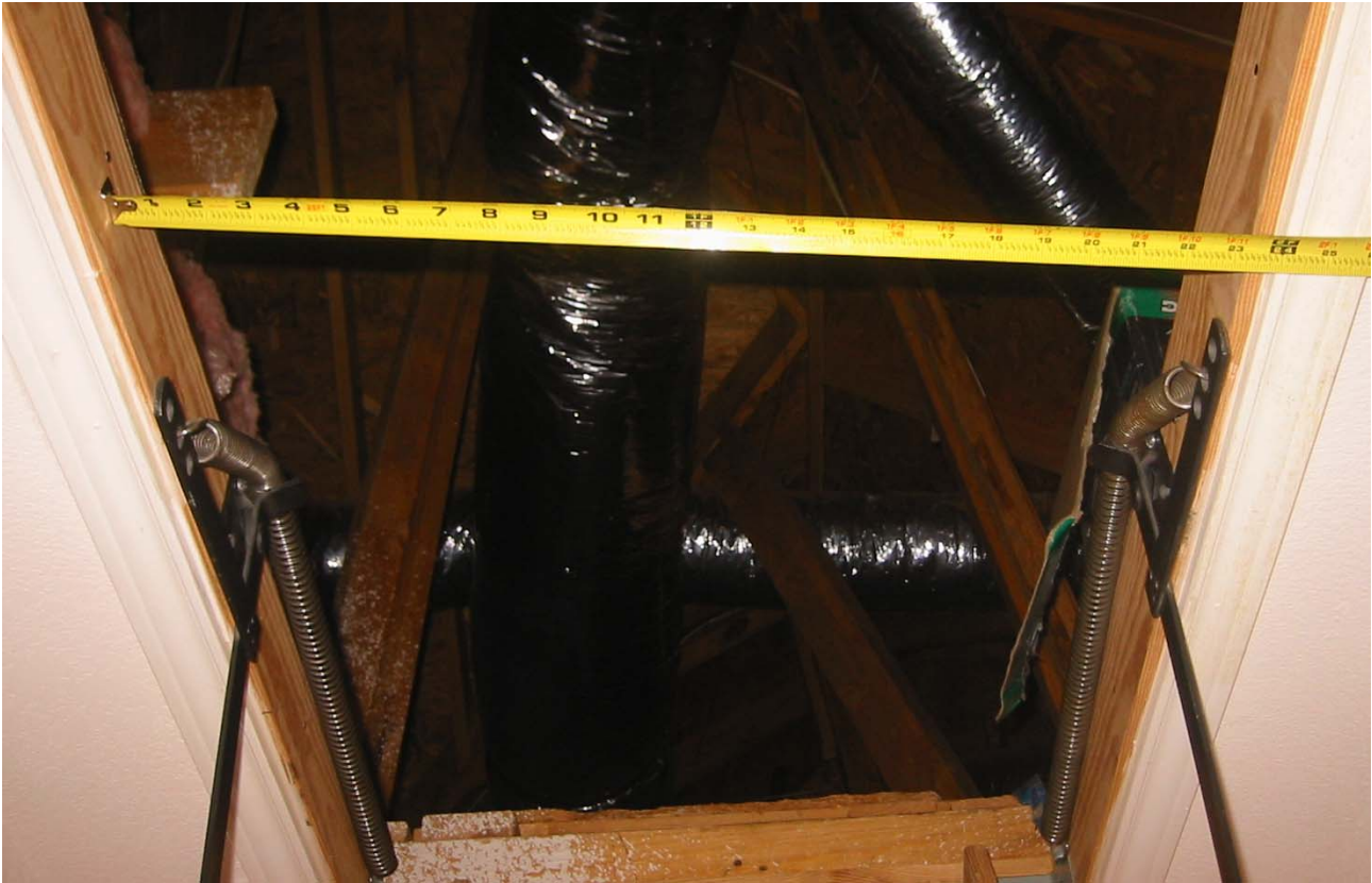
A typical attic pull down ladder for recent new construction that is inadequate for many of today's high efficiency air handler assemblies.
