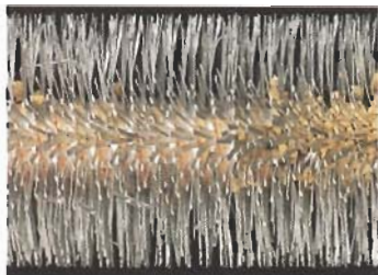
A depth-loading Spine Fin coil has many spines still transferring heat above the accumulated dirt layer.
