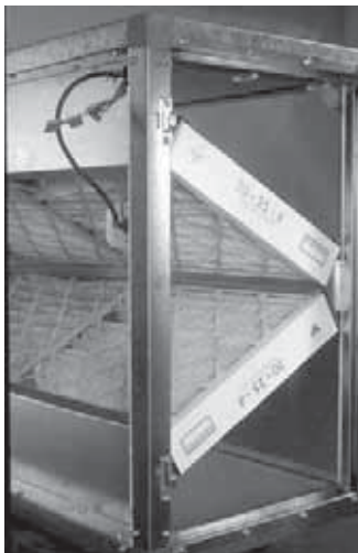
Figure 36. Angled filters increase surface area and lower airside pressure drop
